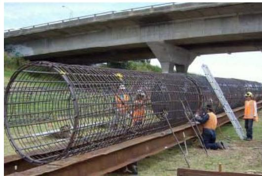
*Welding O-cell Assembly to Reinforcing Cage*
